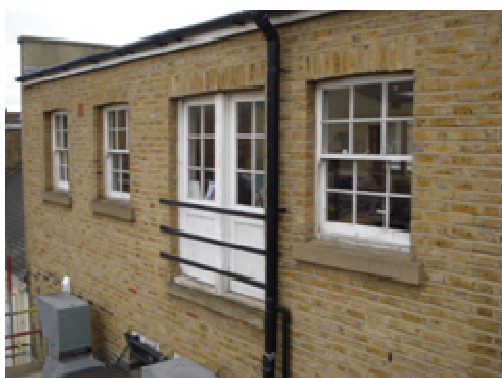
EASTERN ELEVATION OF NUMBER 20 STANNARY STREET TO TOP FLOOR LOOKING SOUTH
