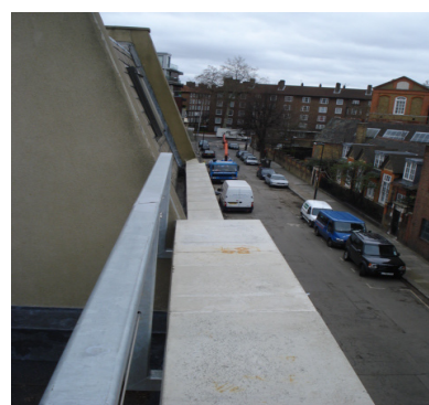
GENERAL VIEW ALONG STANNARY STREET LOOKING SOUTH FROM ROOF OF 22-26 STANNARY STREET
