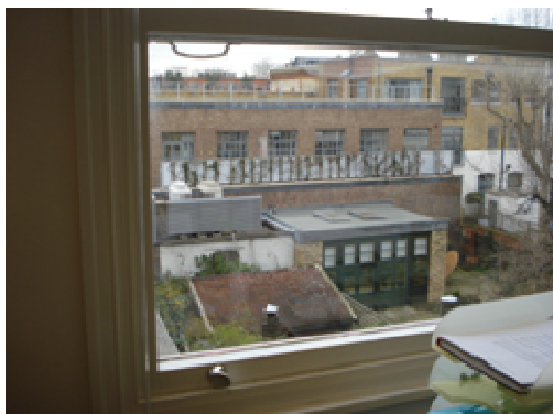
GENERAL VIEW OF EASTERN ELEVATION OF 22-26 STANNARY STREET FROM 184 KENNINGTON PARK ROAD (TOP FLOOR LEVEL) (NOTE ADJOINING BUILDING TO GROUND FLOOR LEVEL IN NEIGHBOURING GARDEN)
